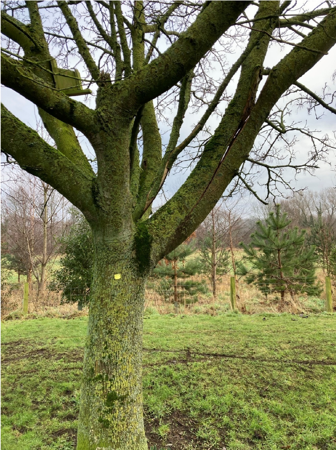
Figure 2 shows tag number 415. There is a large crack in the branch to the right of the tag. This will need removing.
