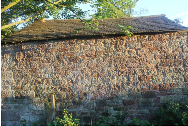
Figure 12: Showing the northern elevation.
